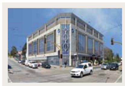
Proposed redevelopment at Epworth Rehabilitation Camberwell
