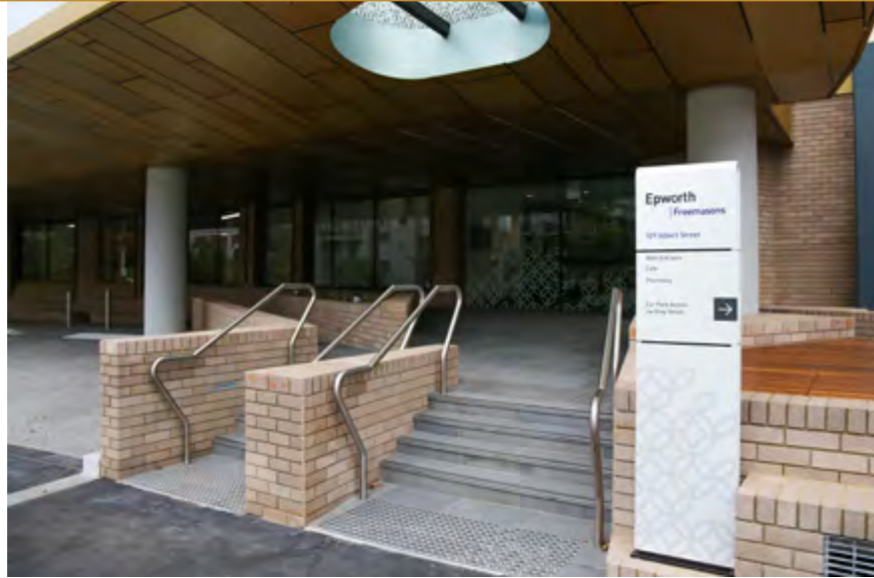
The new entrance at Epworth Freemasons.
