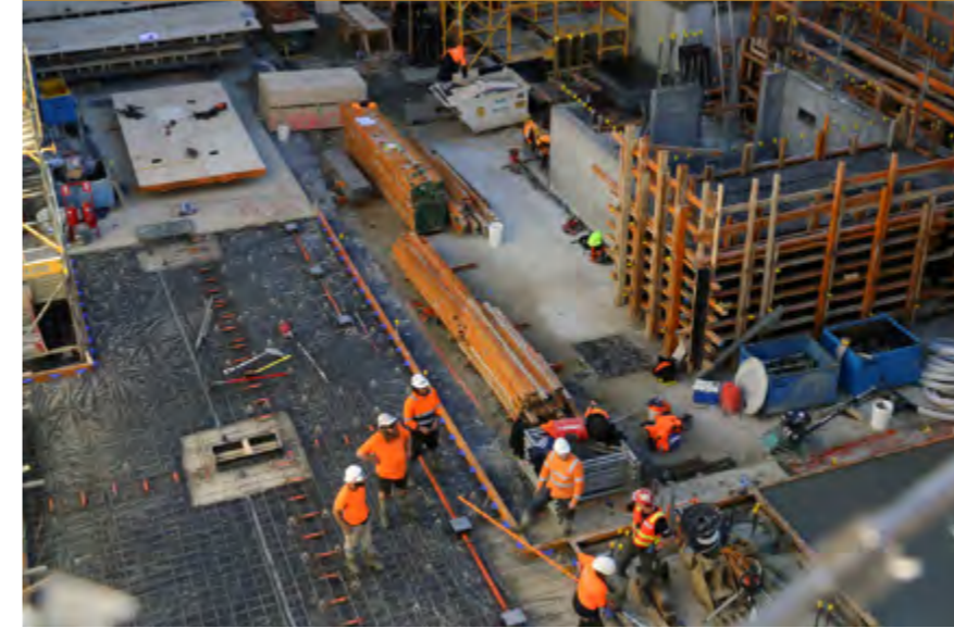
Redevelopment works continue at Epworth Eastern.
